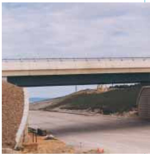
Majors Road bridge
